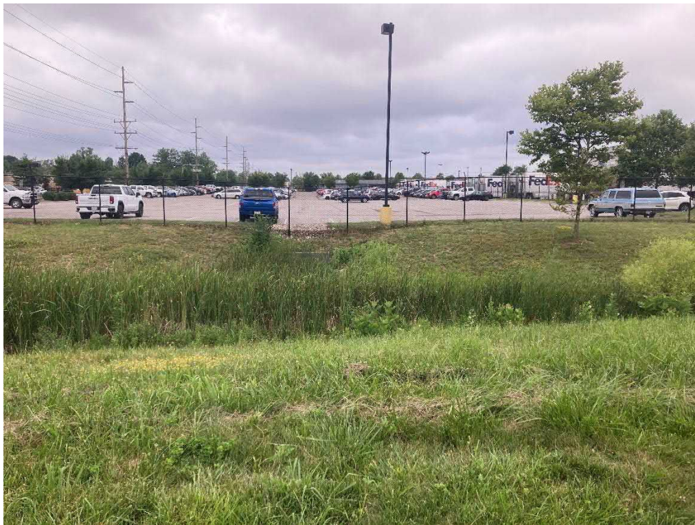
Detention Basin PS-02 facing west on July 8, 2021.
